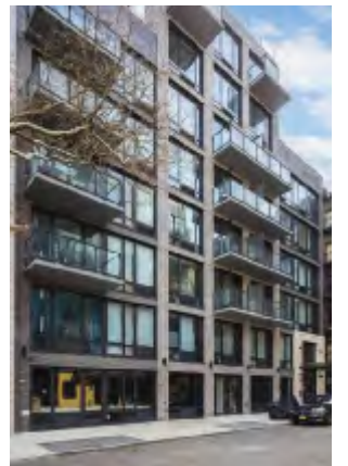
36 25 East 19th Street, Brooklyn Architekt: Issac & Stern Architects Fertiggestellt: 2017 Ziegel: K54, K91 Foto: Dean Kaufman
